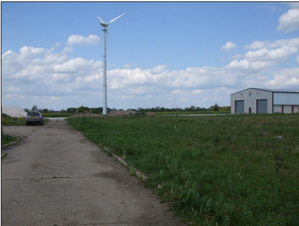
Turbine and agricultural shed
